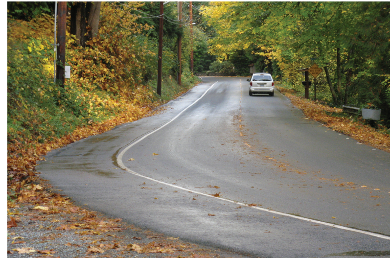
above: paved shoulder
