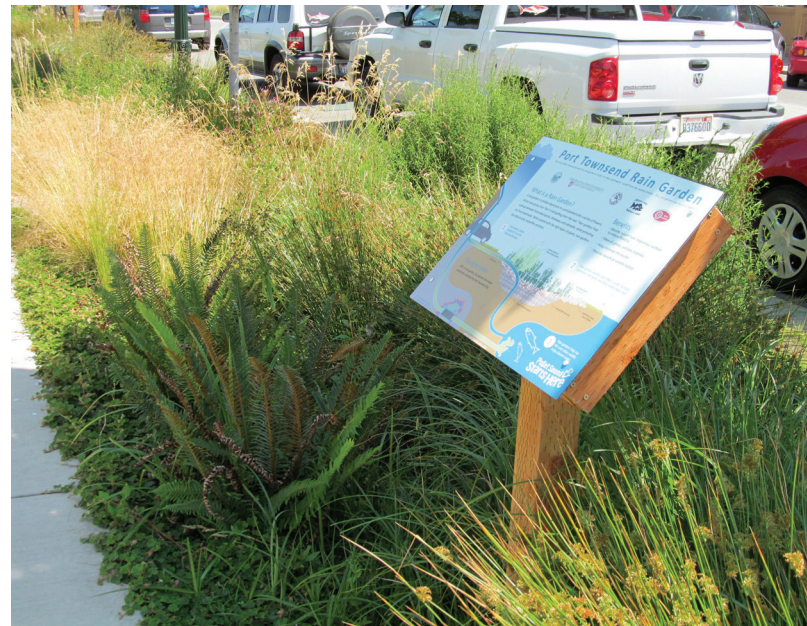
above: bioretention swale
