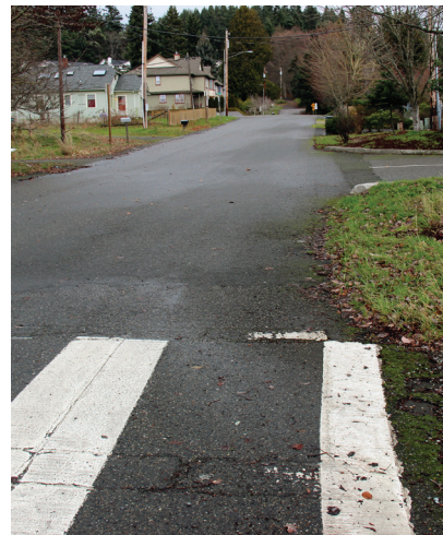
above: existing Iowa Ave
